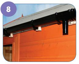
✓ Use a Union Bracket or Angle to join to next gutter length in order to build up a gutter run. Use a Stopend to complete the run.
