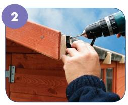
✓ Fix a fascia bracket at the furthest point from the outlet.
