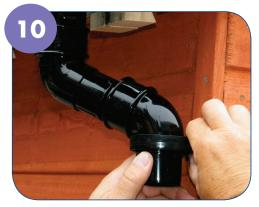
Support downpipes below offset and at maximum intervals of 1 metre.
