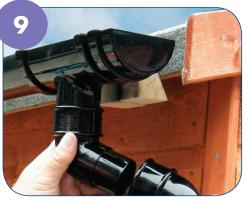
Downpipe installation starts at the outlet. If an offset is required use two Offset Bends with or without a short piece of pipe.
