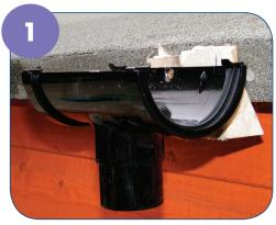
Establish the position of the running outlet and fix the wooden block to the shed. (Wooden blocks are angled dependant on the pitch of your shed roof).
