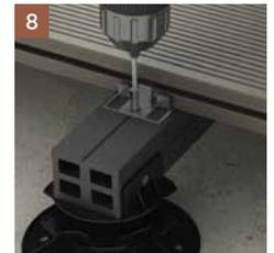
8 Alternative to joists: Composite Decking Keel fixed to height adjustable pedestals using 3 mm x 25 mm stainless steel screws.
