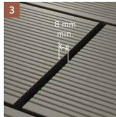
3 Minimum 8 mm end to end gap between butt jointed boards. This gap is important for drainage and to avoid expansion caused by long term immersion.
