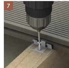
7 Composite Decking stainless steel fixing clip fixed using 3 mm x 25 mm stainless steel screws.
