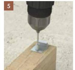
5 Composite Decking stainless steel starter clip fixed using 3 mm x 25 mm stainless steel screws.
